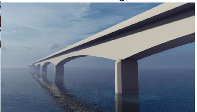
Balanced Cantilever Bridges
