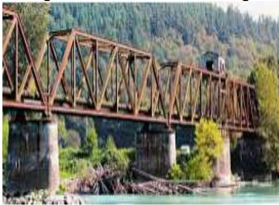
Steel Truss Bridges
