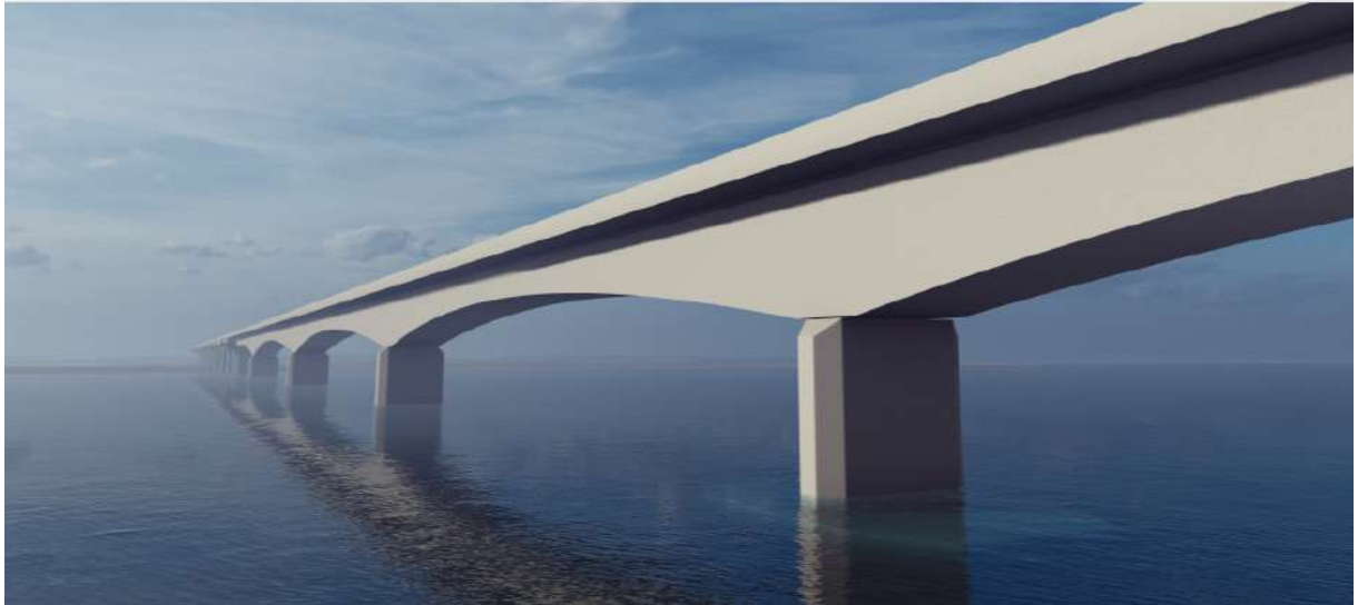
Balanced Cantilever Bridge
