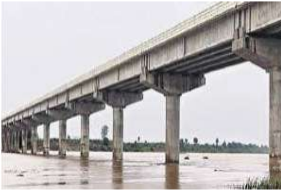
RCC T-Girder Bridges
