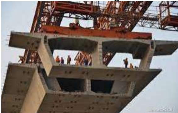
Segmental PSC Box-Girder Bridges
