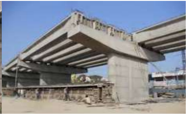
PSC I-Girder Bridges
